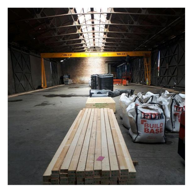
We have a depot at Forth Ports in Leith, this depot will be utilised to prepare the rails for installation. This includes the erecting of portacabins and the temporary construction of a gantry crane, which will be used to handle and prepare the rails for the project.
