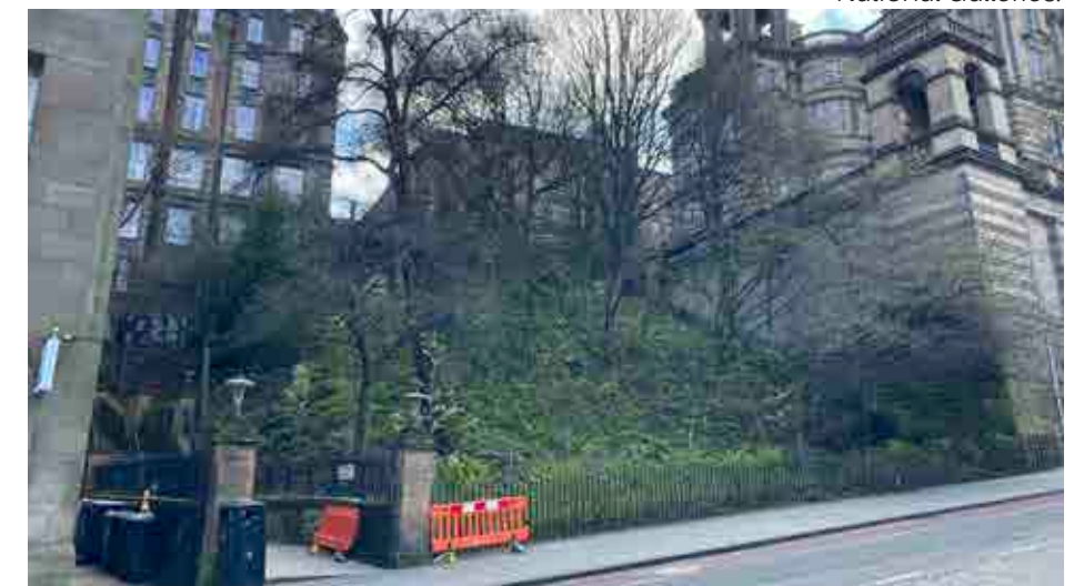
Figure 6.180 The east 'garden' of the Bank of Scotland, next to the News Steps, currently has an overgrown appearance.
