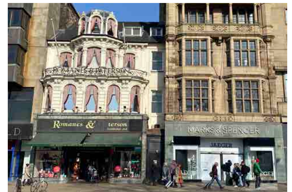
Figure 6.57 61-2 Princes Street (left), remodelled in 1870 for the drapers Romanes & Paterson with a tearoom later added.
