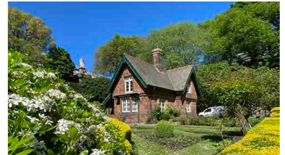
Figure 5.56 Gardener's Cottage was built in 1886 to designs by Robert Morham (2025).
