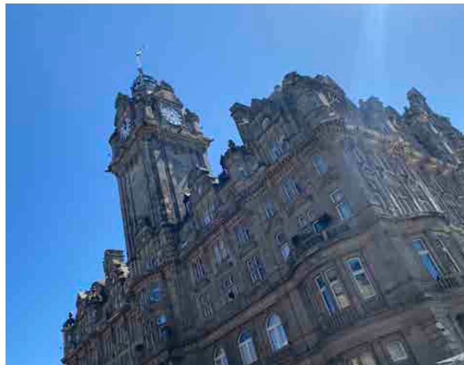
Figure 6.69 The clock tower of the Balmoral Hotel (Former North British Hotel), completed in 1902, has become a recognisable landmark on Edinburgh's skyline.
