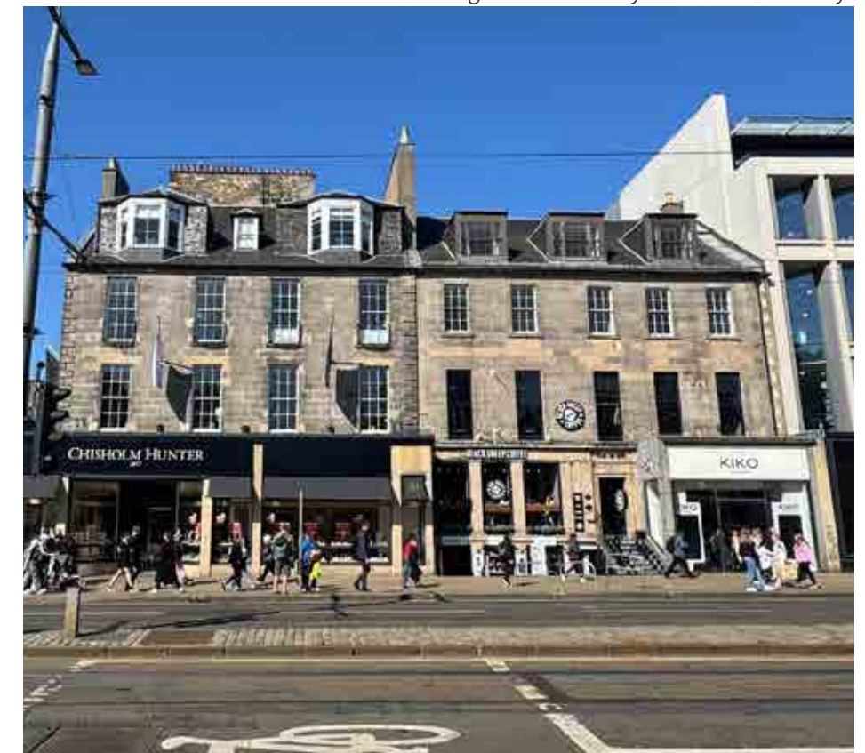
Figure 6.6 Examples of surviving 18th century buildings, with alterations.
