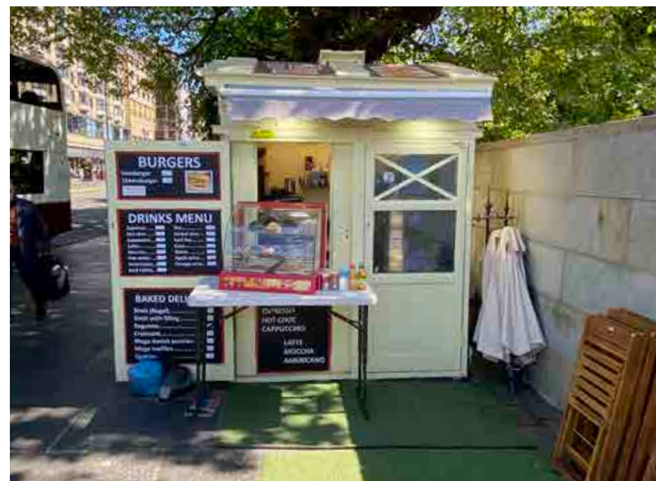
Figure 5.28 Former Police Box (Category B listed) converted into a food outlet.
