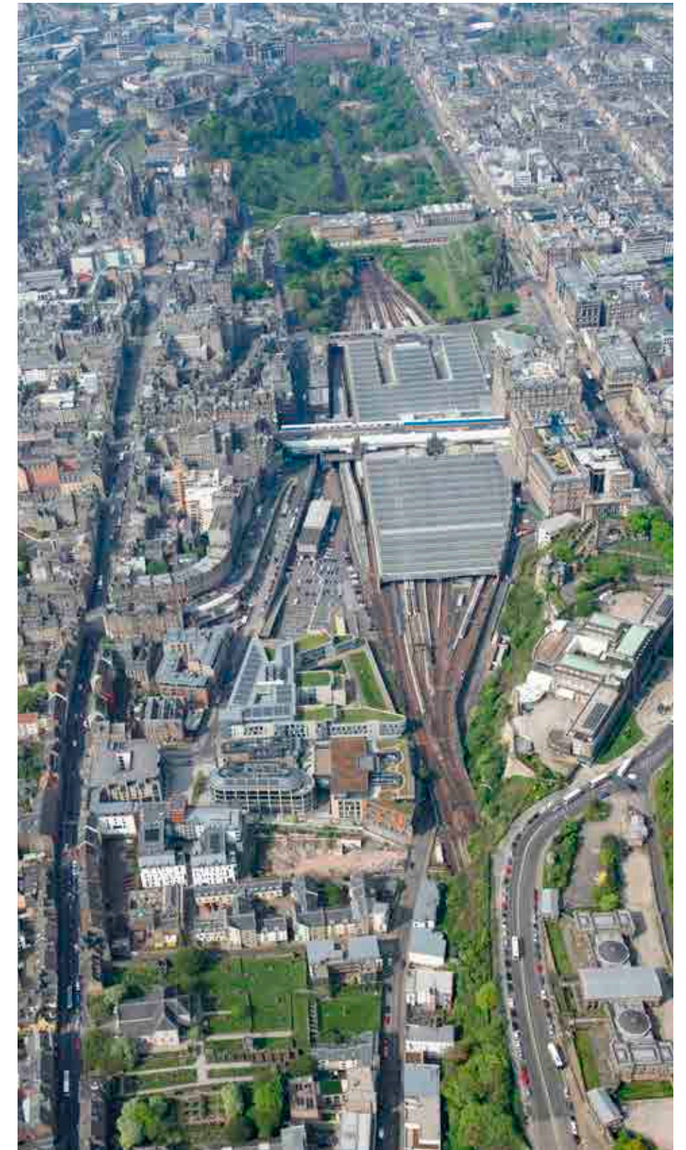
Figure 6.135 Aerial view of the Waverley Valley and Edinburgh Waverley Station with bridges and The Mound connecting the Old and New Towns.
