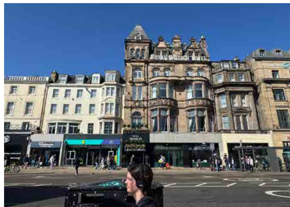
Figure 6.66 Mix of building styles and ages within Block 7.
