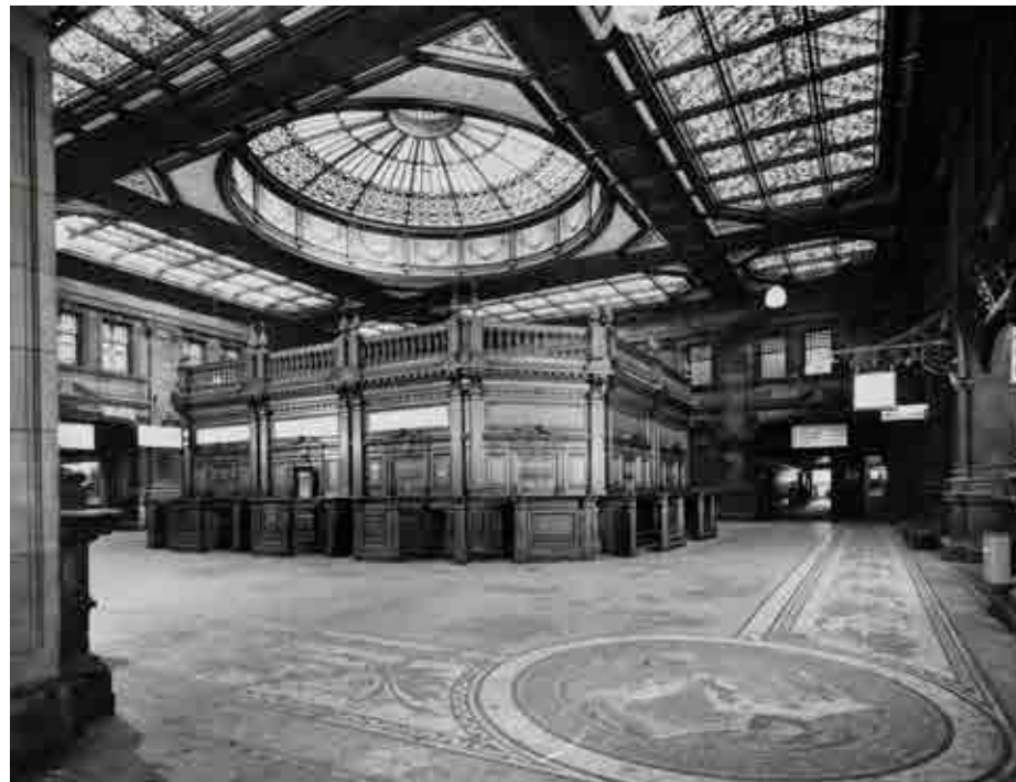
Figure 6.74 Booking Hall in Edinburgh Waverley Station created as part of the 1890s redevelopment (image taken 1969) (SC2661508 © Crown Copyright: HES).
