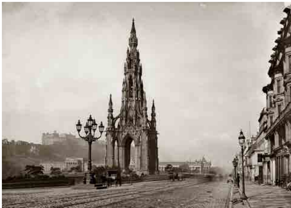
Figure 6.13 Princes Street and the Waverley Valley are associated with past lives and events (City of Edinburgh Council - Libraries www.capitalcollections.org.uk ).
