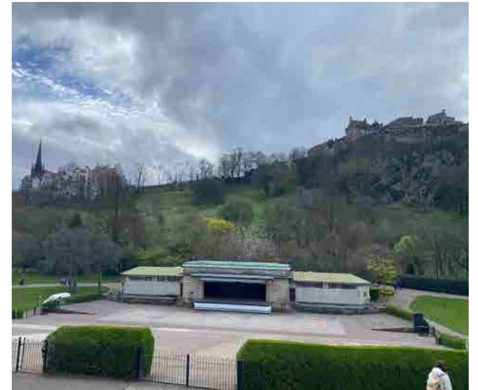
Figure 6.171 Ross Bandstand in West Princes Street Gardens.
