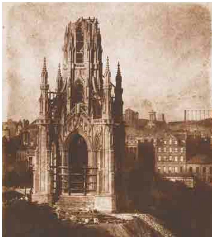
Figure 4.6 Sir Walter Scott Monument under construction (City of Edinburgh Council - Libraries www.capitalcollections.org.uk ).
