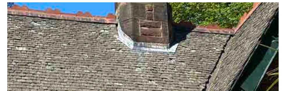
Figure 5.15 Slate roof of Gardener's Cottage.
