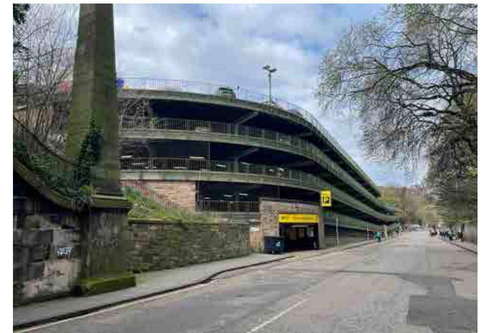
Figure 6.23 Castle Terrace Car Park is located on the edge of the Study Area and represents Scotland's first multi-storey car park.
