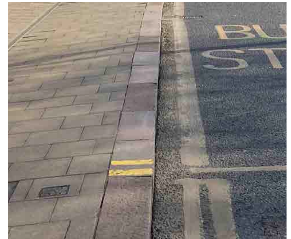
Figure 5.25 Stepped kerbs marking the delineation between the road and pavement.
