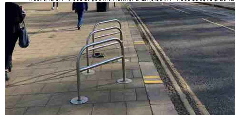
Figure 6.141 Public bike racks located on the north pavement at the west end of Princes Street.
