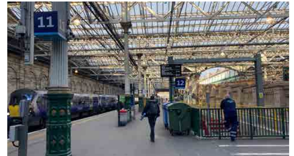
Figure 6.71 Interior of Edinburgh Waverley Station, much of the current station fabric dates from the 1890s reordering including the ridge-and-furrow glass roof.
