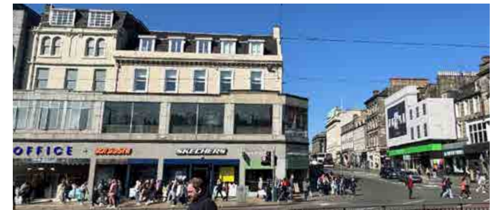
Figure 6.48 78-79 Princes Street, Block 4 is bookended by surviving 18th century buildings with alterations.
