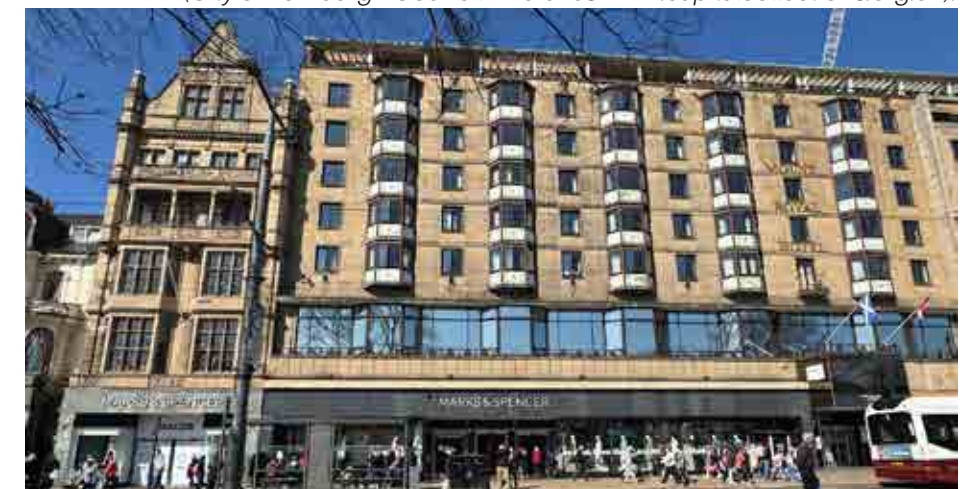
Figure 6.52 Marks & Spencer's, 54 Princes Street, extends into the Category B listed 60 Princes Street (left).
