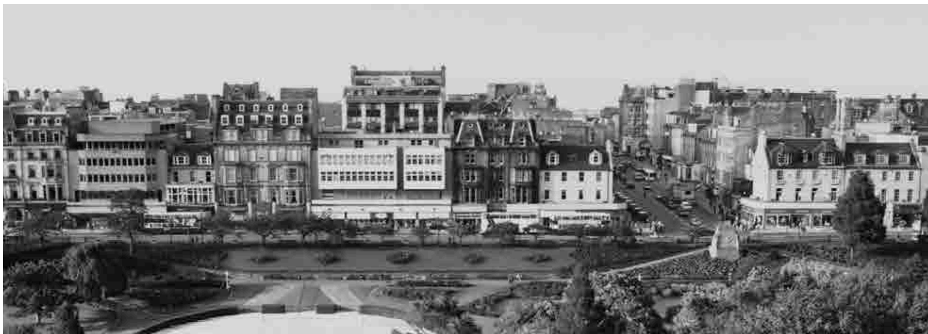
Figure 6.41 C.1980 view, over West Princes Street Gardens, towards the east end of Block 3. The recently demolished Princes Street Panel building (Nos. 107-108) can be seen to the left of the frame (SC 2656612 © HES).
