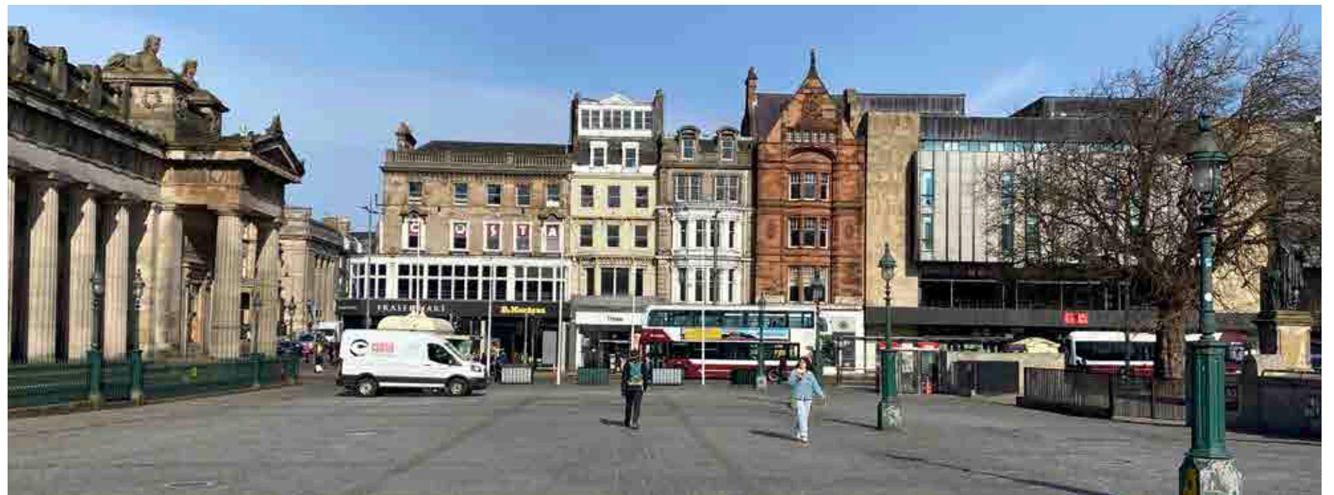
Figure 6.108 View to Princes Street from The Mound showing buildings faced with various materials.
