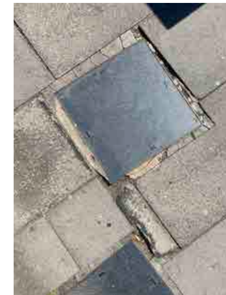
Figure 6.113 Examples of damaged paving on Princes Street (left) and poor patch repairs (right).
