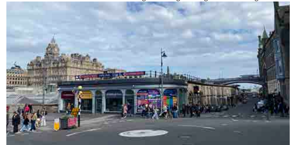
Figure 6.72 The oldest part of the station survives as the Travel Hub, on the corner of Waverley Bridge and Market Street which reused parts of an earlier station building. Along Market Street are former warehouses and offices dating from the 1890s reordering.
