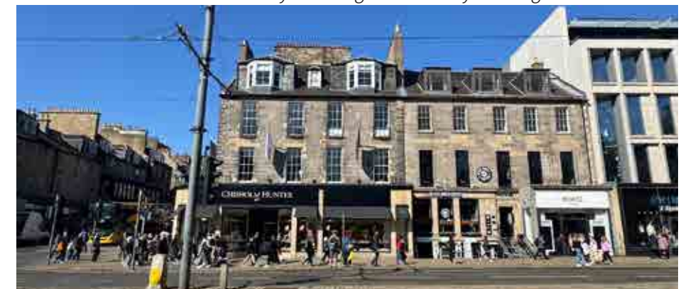
Figure 6.49 94-98 Princes Street, Block 4 is bookended by surviving 18th century buildings with alterations.
