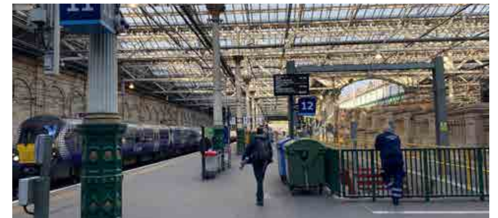
Figure 6.9 Edinburgh Waverley Station, the 'Gateway to Scotland', is a busy interchange of arrivals and departures.
