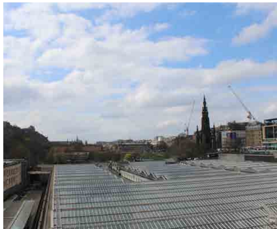
Figure Ap1.34 View 42, Princes Street Gardens CMP
