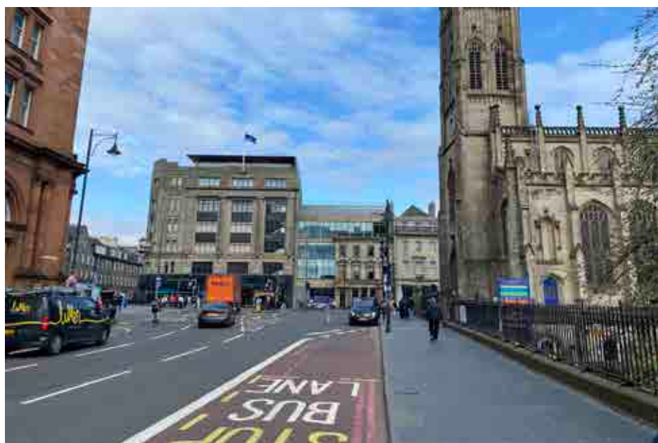
Figure 6.24 View from Lothian Road looking north to Block 1.
