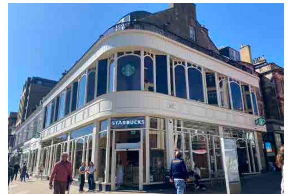
Figure 6.37 118-Princes Street, with a glazed timbered framed extension, now houses a Starbucks and has been recently restored and refitted.
