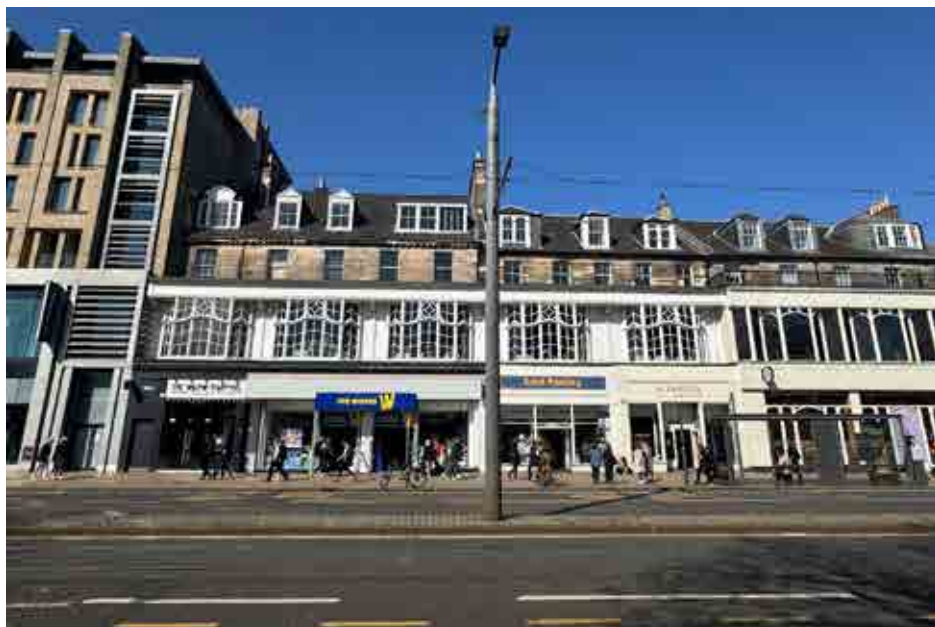
Figure 6.35 118-120 Princes Street with glazed timber framed extensions, associated with the rise of tearooms in the early 20th century.
