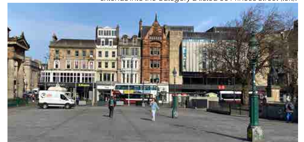
Figure 6.53 West end of Block 5 showing a range of architectural styles (Nos. 64-77), ranging from the 18th to 20th centuries.
