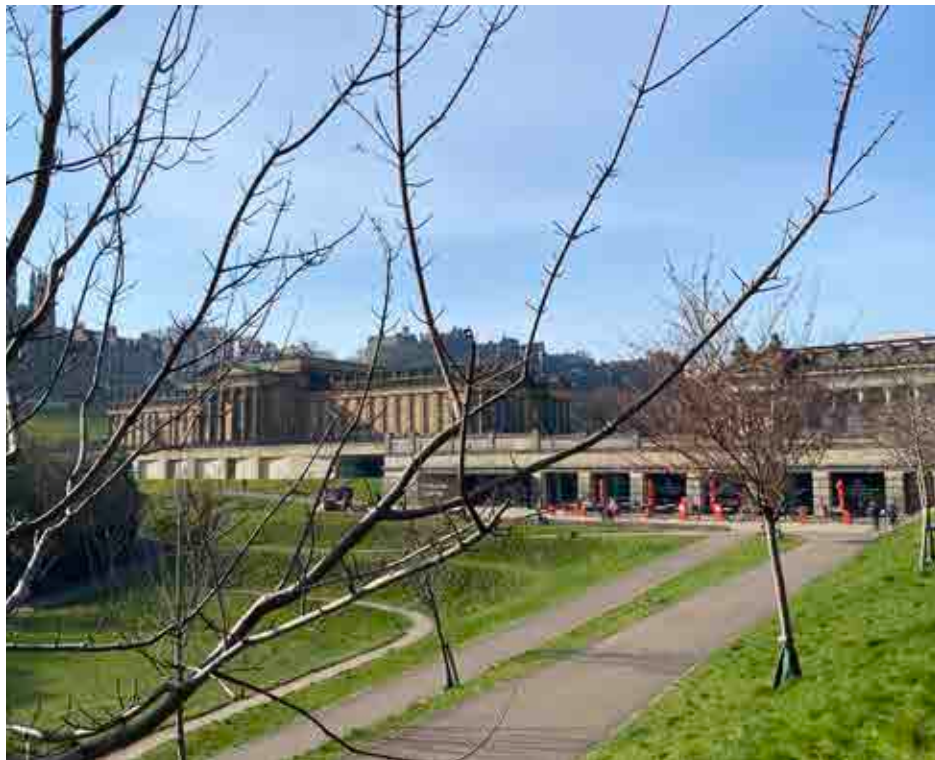
Figure 6.84 View from East Princes Street Gardens to the Royal Scottish Academy and the National Gallery of Scotland.
