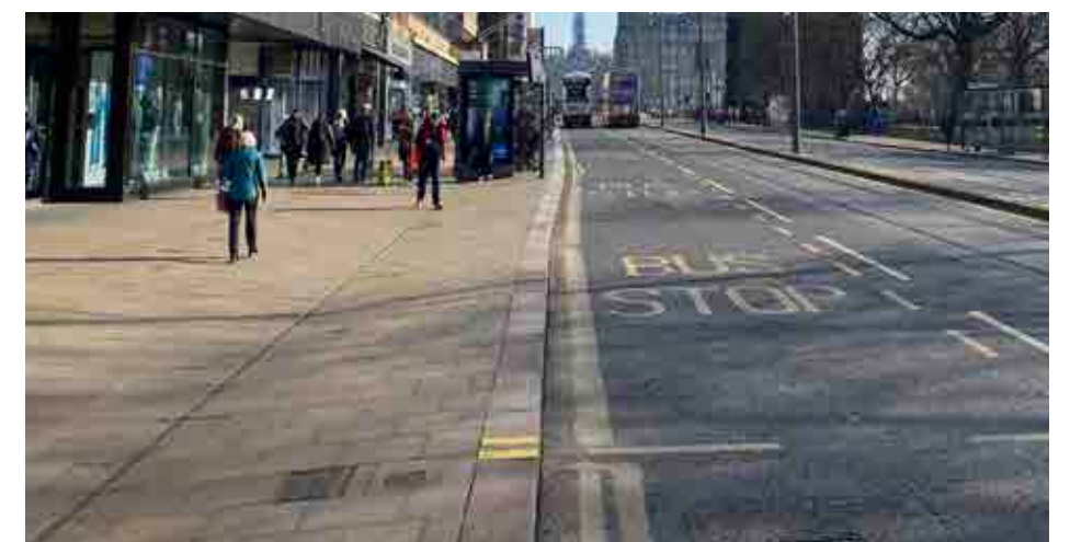
Figure 5.21 2025 image showing widened pavement laid with concrete slabs and tarmacked road surface with tram lines.
