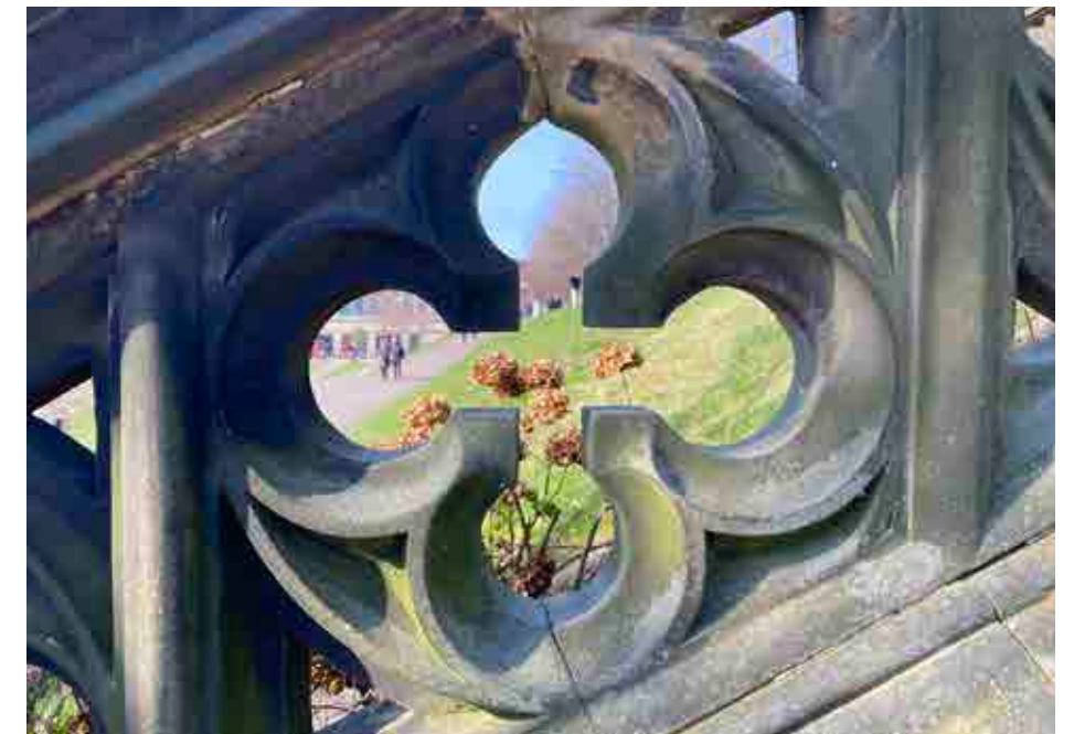
Figure 6.15 Detail view of Cousin's 'gothic character' stone balustrade within East Princes Street Gardens.
