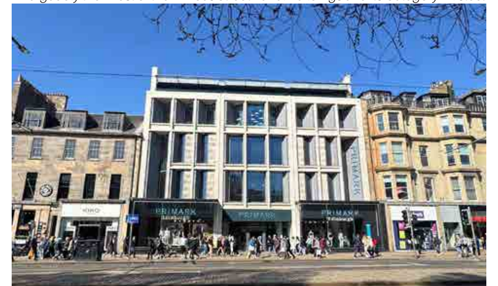
Figure 6.47 Primark, 91-93 Princes Street, built in 2010 replacing a Princes Street Panel building on the site.
