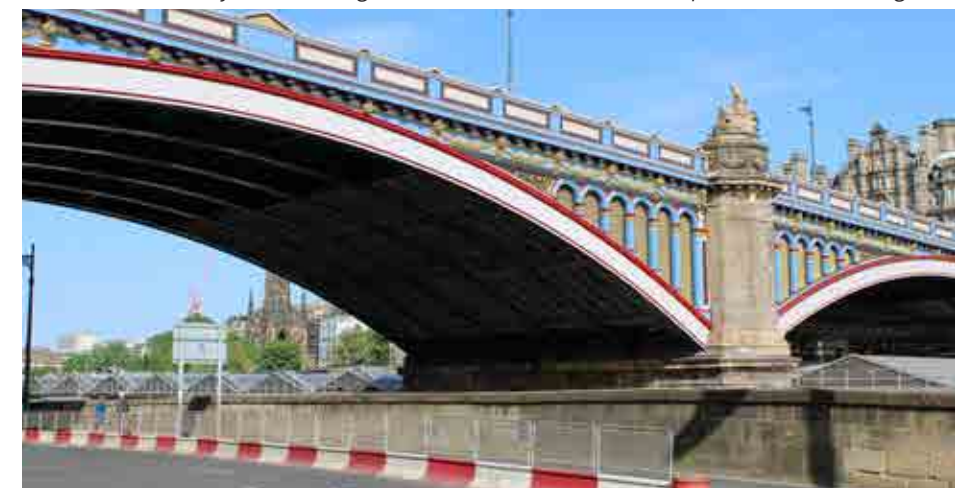
Figure 6.87 View from Market Street to the recently conserved North Bridge, this version of the bridge dates from the 1890s reordering of the station.
