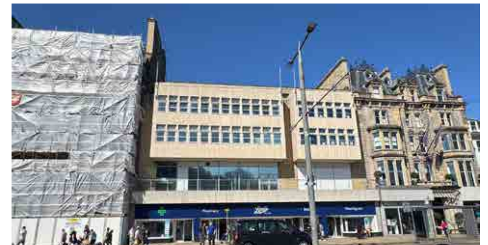
Figure 6.39 An unlisted Princes Street Panel building at Nos. 101–103. To the left is Nos. 104–108 covered in scaffolding and undergoing redevelopment.
