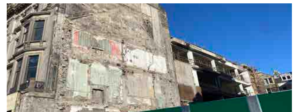
Figure 6.20 This gable has been temporarily exposed as part of consented development works on Princes Street, revealing earlier phases, including a former gable that has been incorporated into later fabric.
