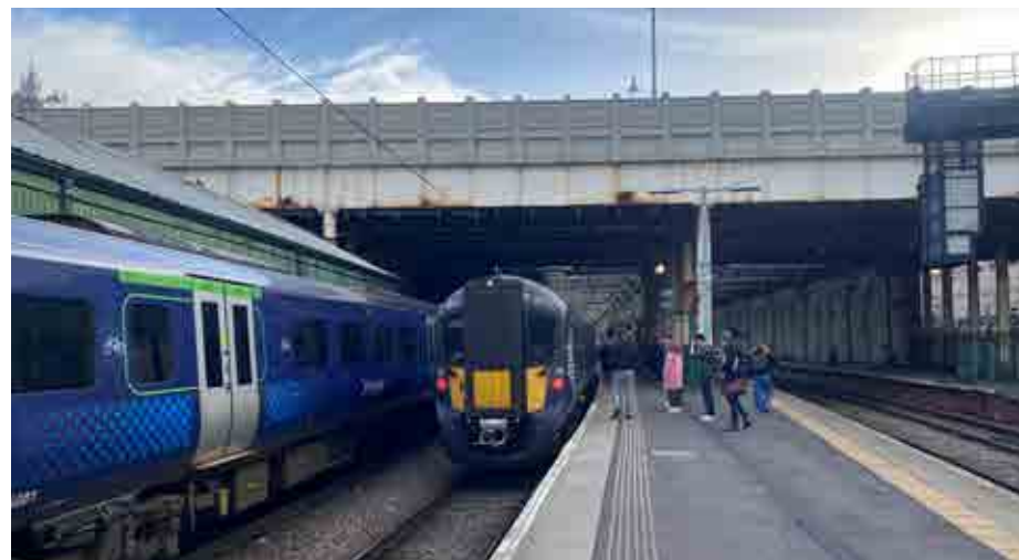
Figure 6.78 View from a platform into the station with Waverley Bridge above, note the fibreglass cladding which conceals the appearance of the bridge and restricts views.
