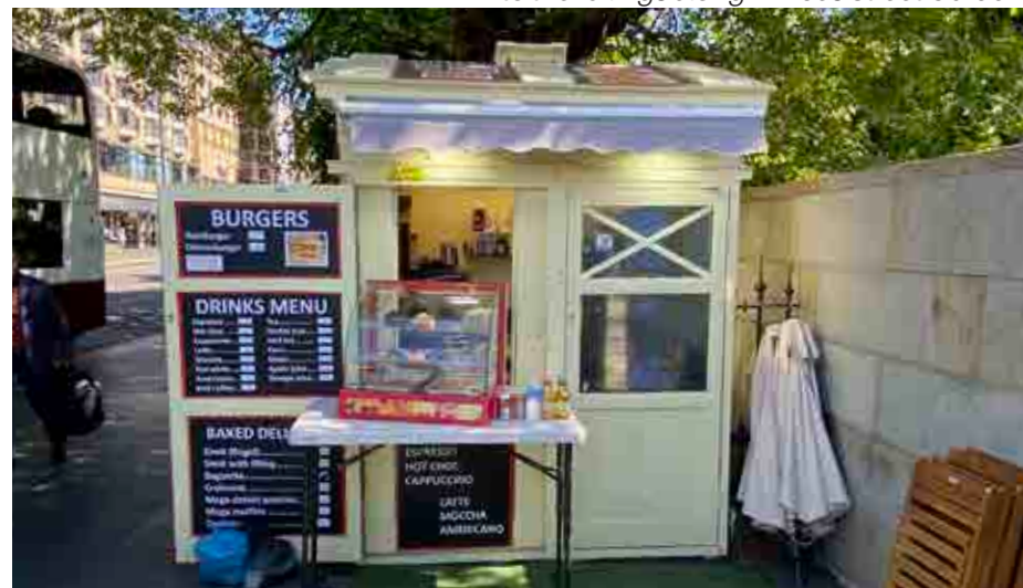
Figure 6.138 Former Police Box, Category B listed repurposed into a food and drink outlet.
