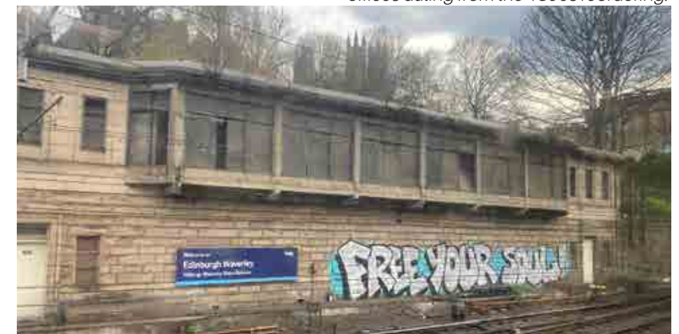
Figure 6.73 A bespoke signal box made from reconstituted stone and concrete, built 1936.
