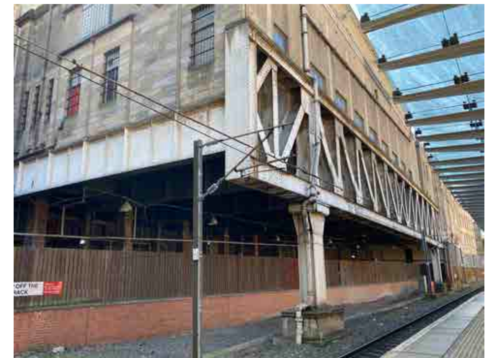
Figure 6.81 Cantilevered steel frame supporting former warehouses and offices along Market Street (31-39 Market Street), seen from within station and southernmost platforms.
