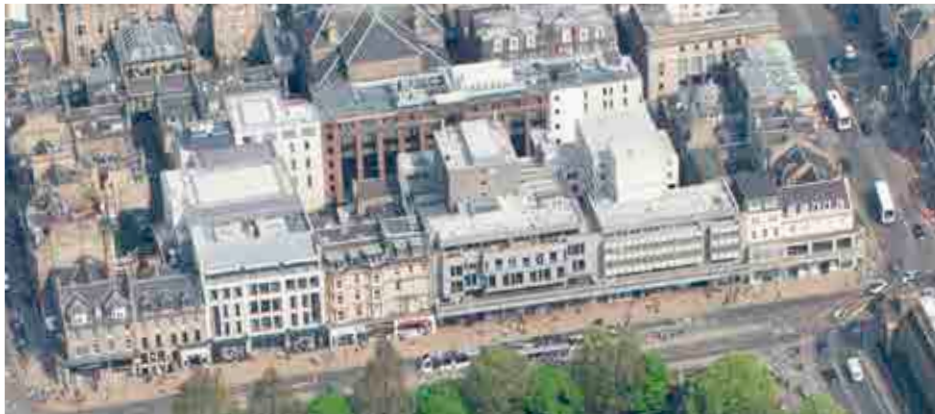
Figure 6.50 Block 4, showing 80-83 and 84-87 Princes Street with taller set back elements, featuring blank façades, visible from elevated vantage points.
