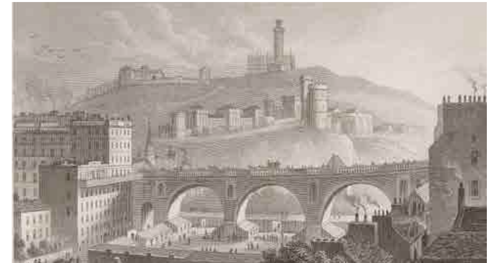
Figure 6.85 1829 view of Mylne's North Bridge (City of Edinburgh Council - Libraries www.capitalcollections.org.uk ).
