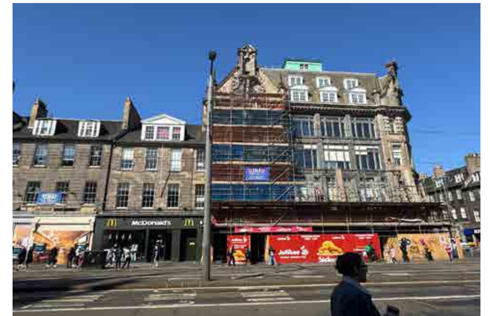
Figure 6.26 Charlotte House dominating the corner plot at the east end of Block 1.
