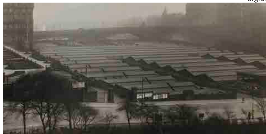
Figure 5.41 1938 Waverley Station after its second major reordering in the 1890s (City of Edinburgh Council - Libraries www.capitalcollections.org.uk ).
