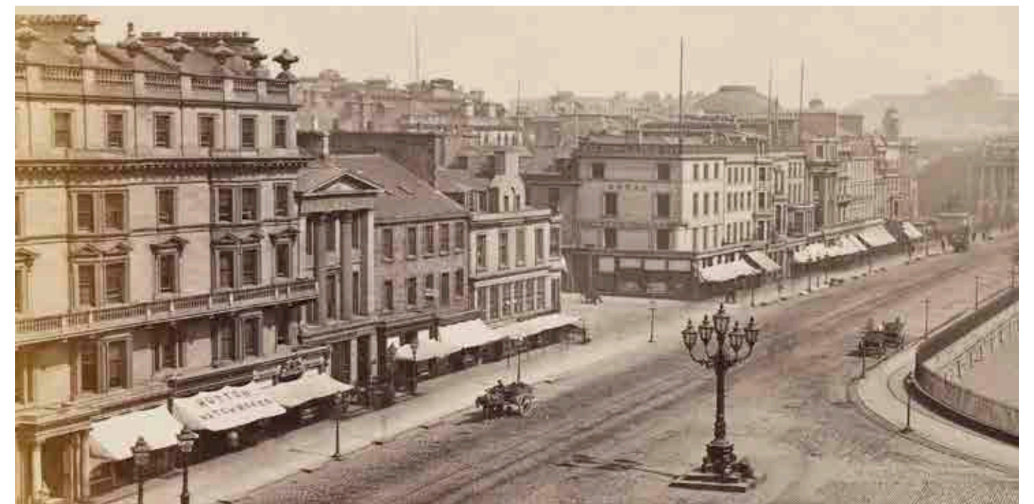
Figure 4.12 1880 East end of Princes Street showing redevelopment of eighteenth century buildings (City of Edinburgh Council - Libraries www.capitalcollections.org.uk ).
