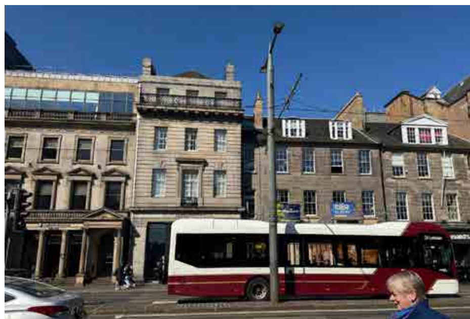
Figure 6.25 Only two buildings in block 1 date from the original construction phase, 137-138 and 139-140 Princes Street, which can be seen to the right of this image.
