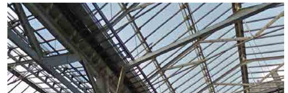
Figure 5.16 Glazed roof of Waverley Station.
