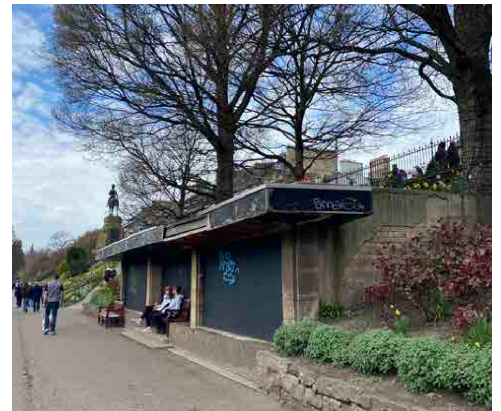
Figure 6.173 Dilapidated listed shelters in West Princes Street Gardens.
