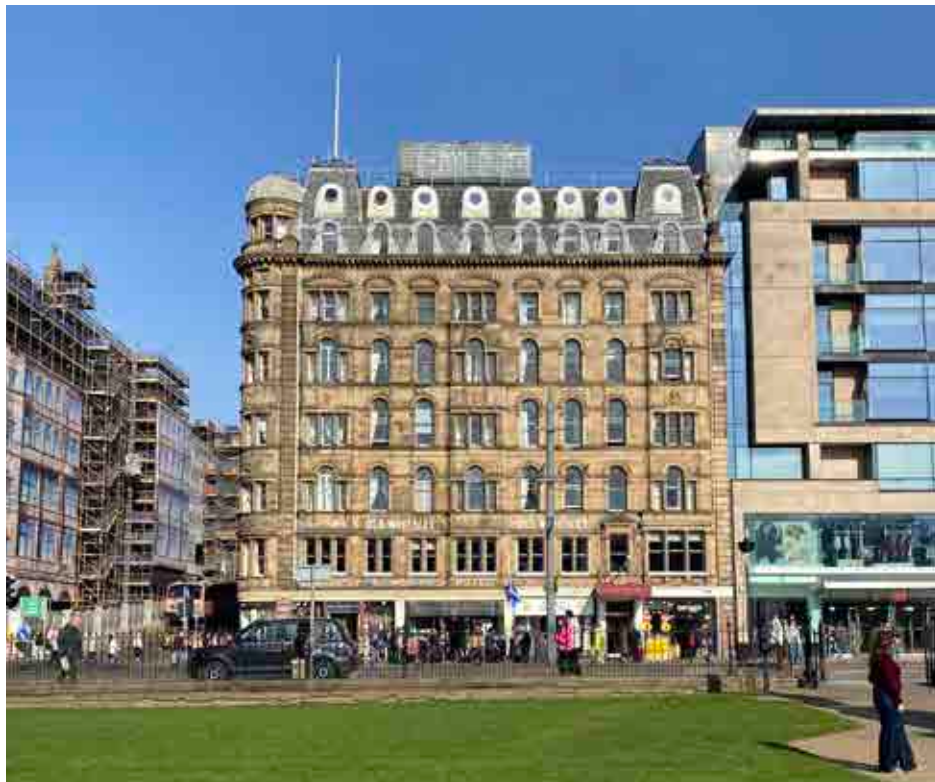
Figure 6.58 Old Waverley Hotel, 42-46 Princes Street, the oldest surviving building within Block 6.
