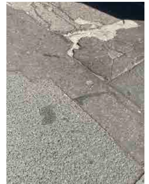
Figure 6.113 Examples of damaged paving on Princes Street (left) and poor patch repairs (right).
