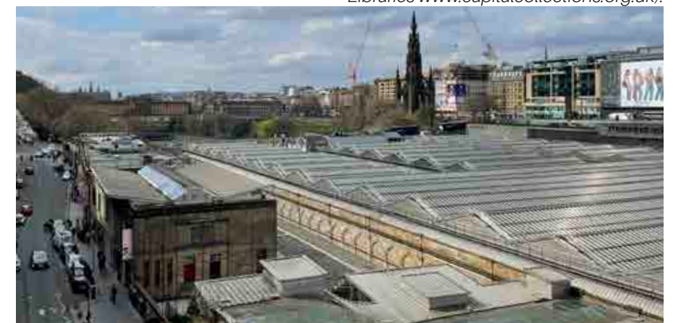
Figure 5.42 2026 view from North Bridge over the glazed roof of Edinburgh Waverley Station.
