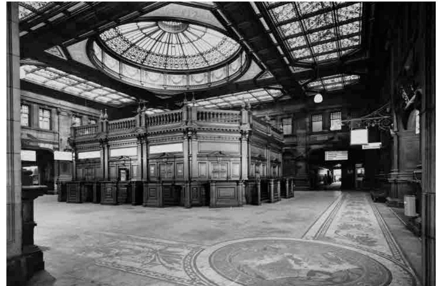
Figure 4.13 Booking Hall in Edinburgh Waverley Station created as part of the 1890s redevelopment (image taken 1969) (SC2661508 © Crown Copyright: HES).
