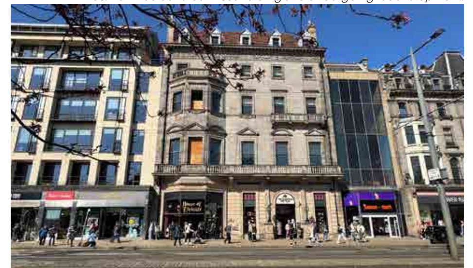
Figure 6.40 112 Princes Street was built for the Scottish Conservative Club, the facade was retained in 1978–81 when it was converted to a Debenhams, consent has been granted for its conversion into a hotel with associated uses.
