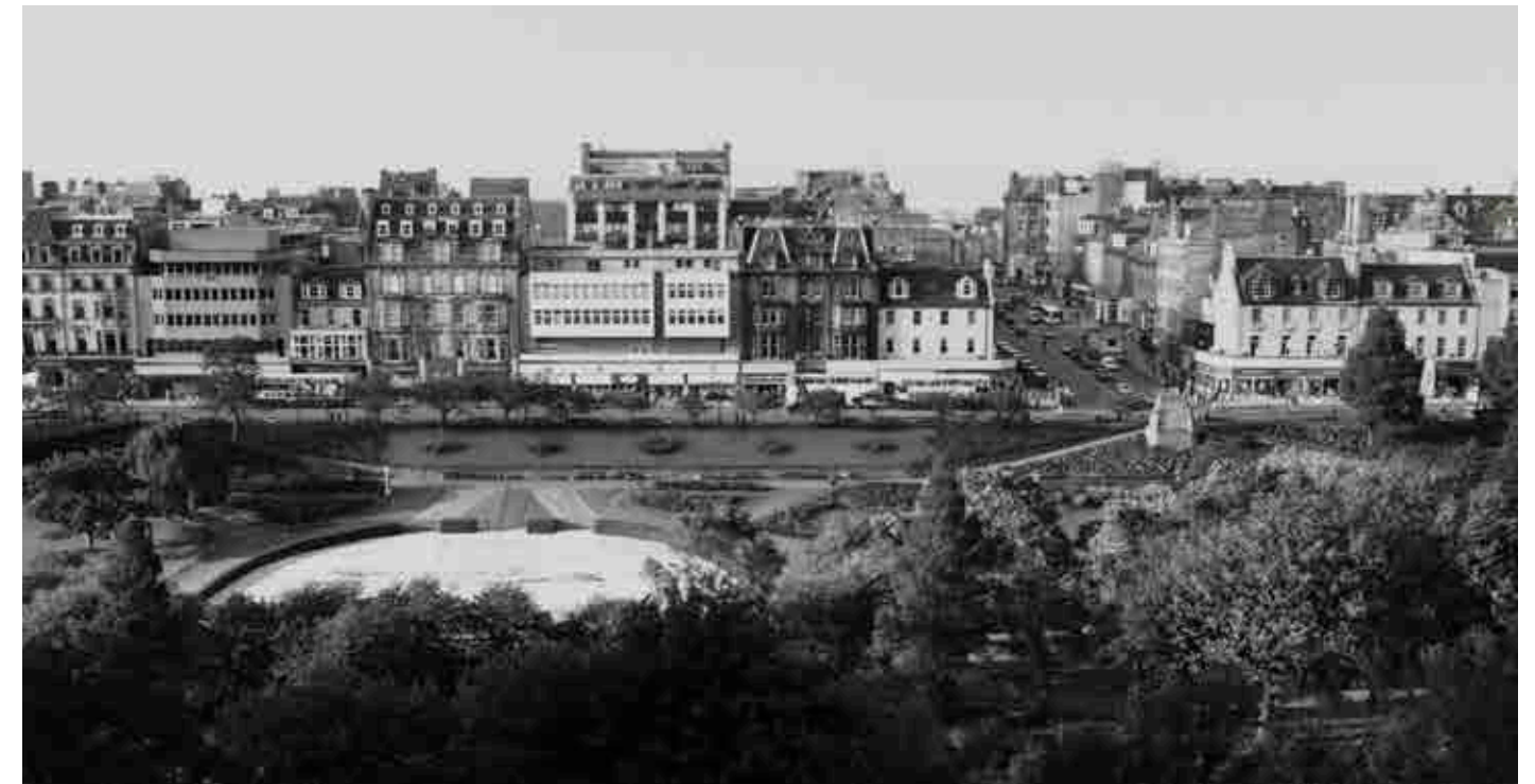
Figure 4.17 C. 1980 view towards Princes Street showing its architectural variety with West Princes Street Gardens and seating for the Ross Bandstand in the foreground (SC 2656612 © HES).
