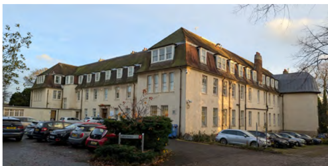
Unlisted Heritage Asset
