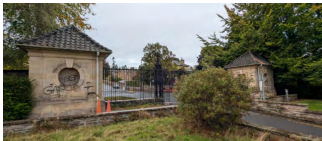
Category B Listed On Buildings at Risk Register
