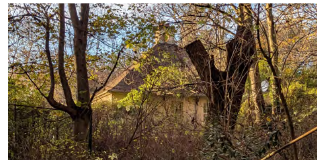
Unlisted Heritage Asset
