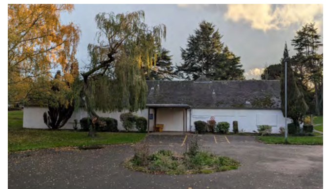
There is a high level of carriageway on the site, and some parts of the site lack footways entirely
