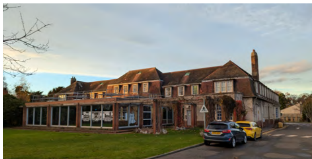
Unlisted Heritage Asset
