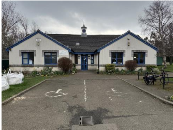
1 Front view of building entrance, including bike racks and accessible parking
