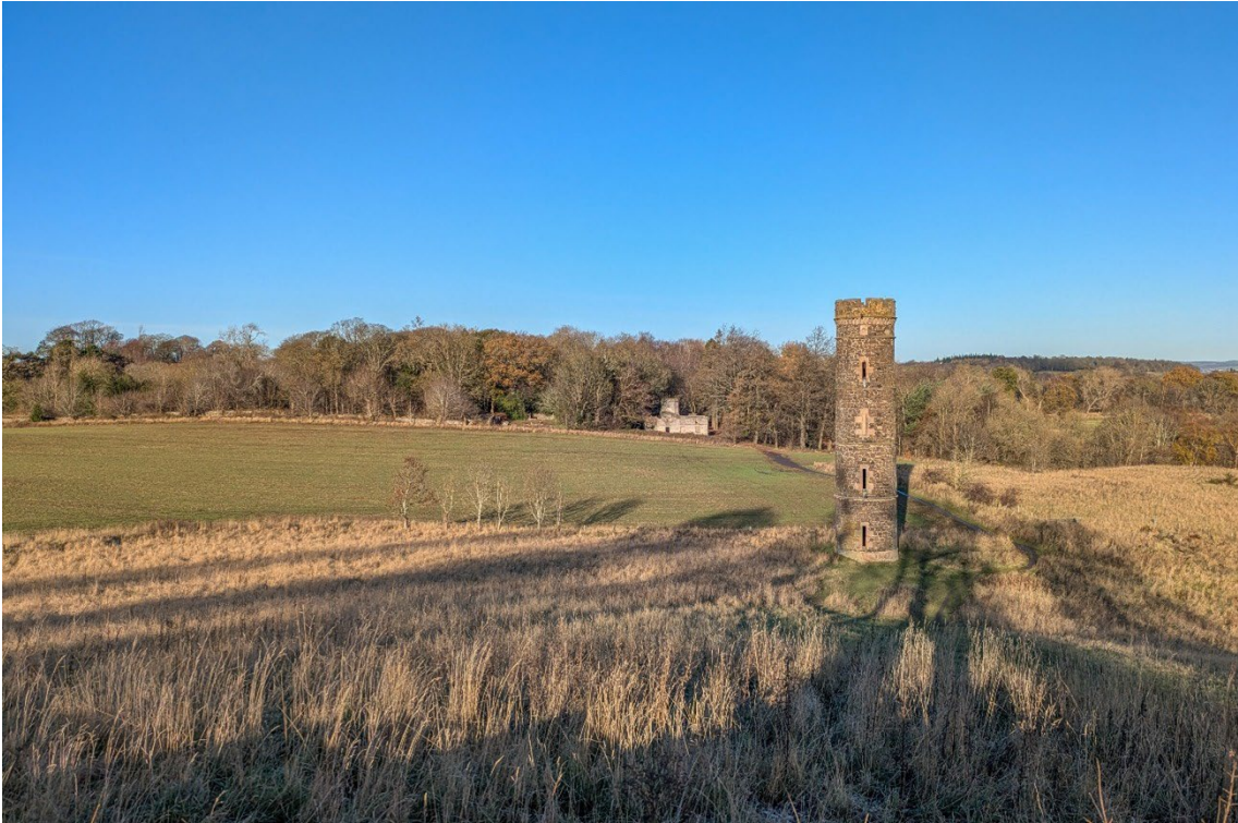
Figure 2.5: The Cammo Water Tower forms a distinctive landmark on the skyline rising above rectilinear fields, with woodland seen beyond
