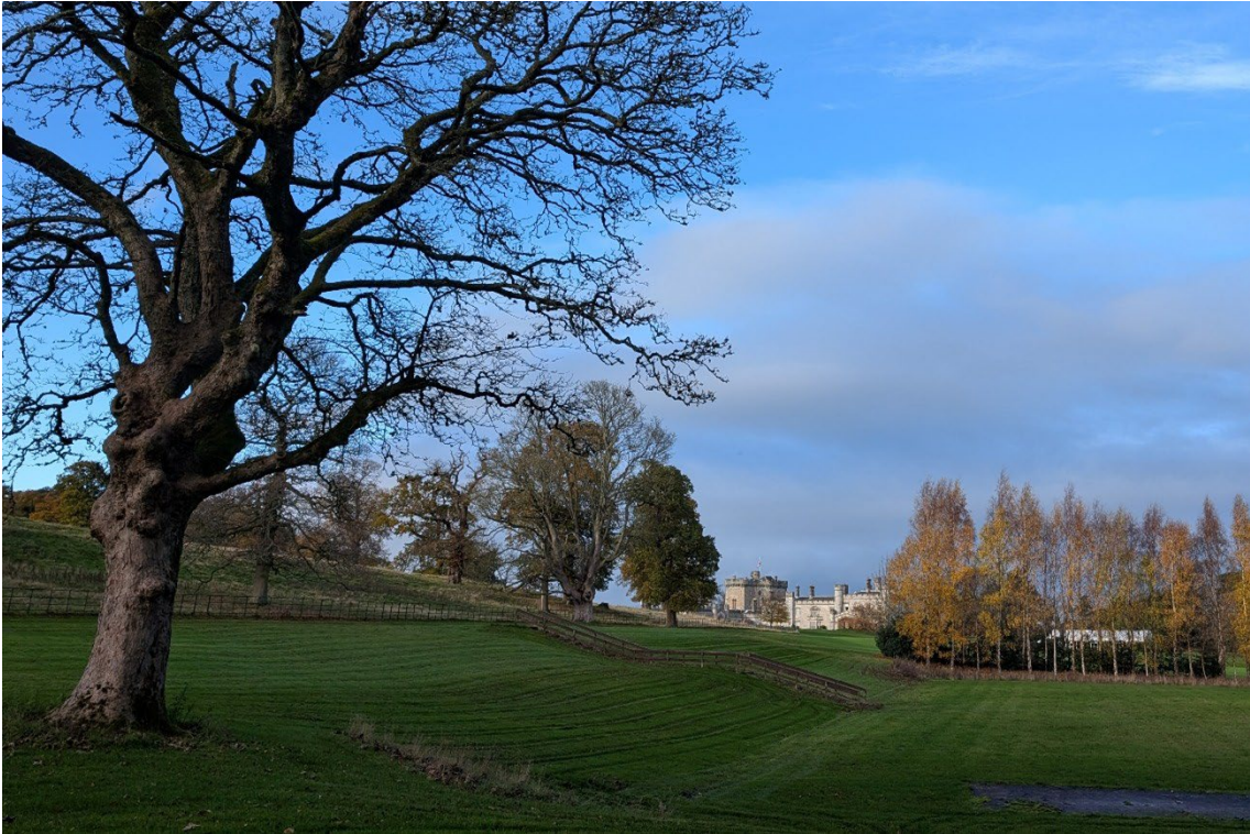
Figure 2.7: The Listed Dundas Castle is set within a context of well-managed farmland with woodland and shelterbelts
