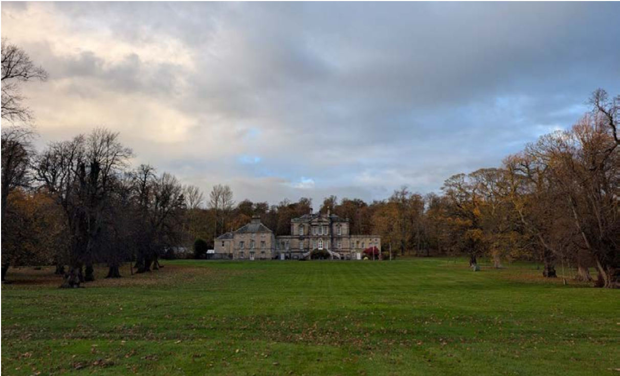
Figure 3.78: Drum House is set amidst dense woodland and lawns lined by avenue trees
