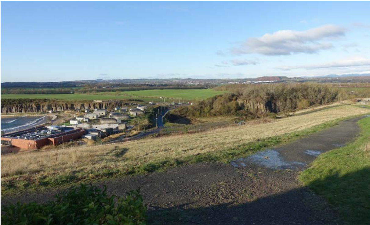
Figure 3.131: View west from the edge of Ratho village, with part of Lost Shore Surf Resort set within the former Craigpark Quarry in the middle distance
