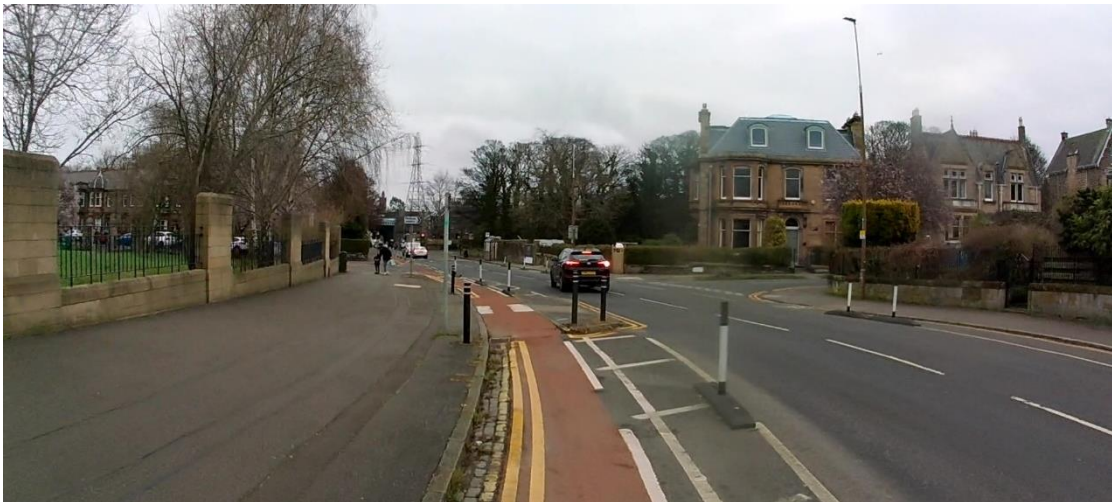
Figure 3-5: Segregated Cycle Lanes Integrated Well with Existing Permanent Infrastructure on Duddingston Road
