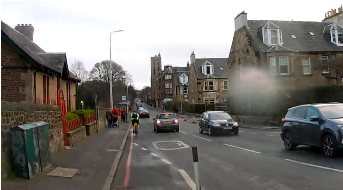
Figure 3-3: Road Markings Indicating the End of the Segregated Cycle Lane
