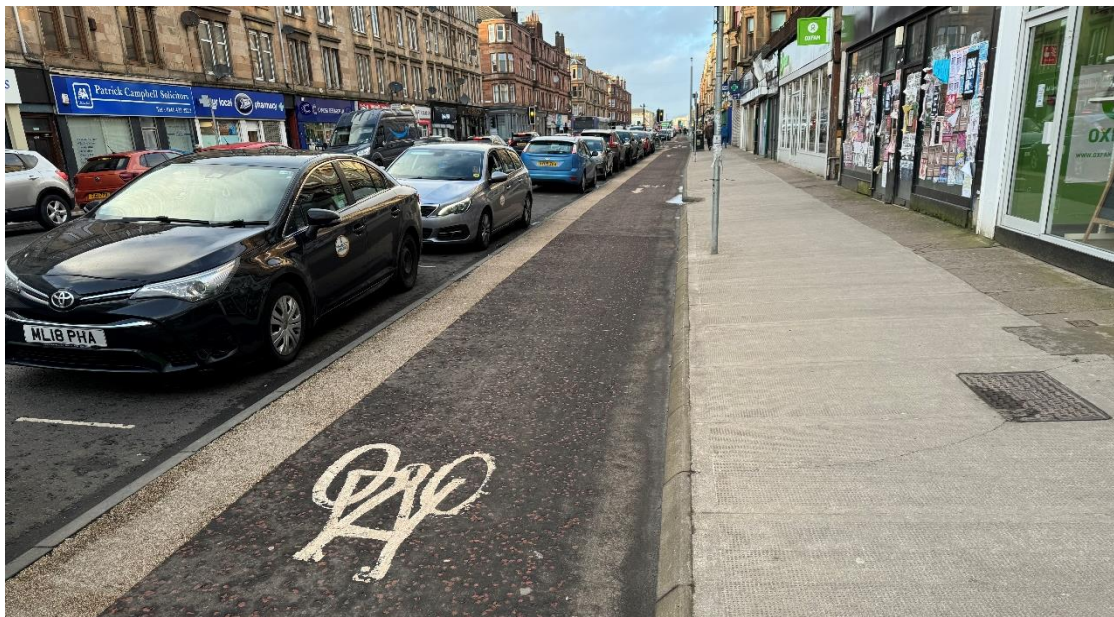
Figure 8-1: Stepped Cycleway at Intermediate Level with a Marked Buffer Zone (Victoria Road, Glasgow)
