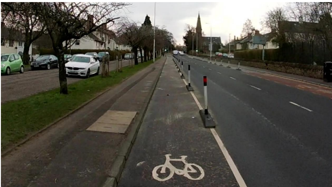
Figure 2-1: Example of a Segregated Cycle Lane with Lane Defenders on Gilmerton Road
