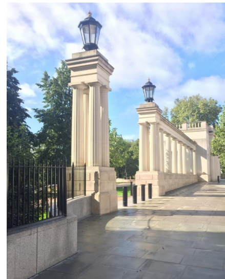
FIGURE 8. VSBs 'DISGUISED' INSIDE BOUNDARY WALL WITH RAILINGS AT GREEN PARK, LONDON
