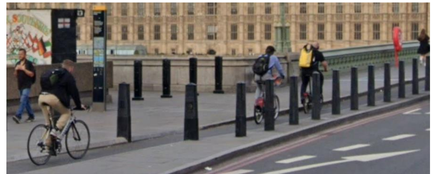
FIGURE 10. 1200MM HVM AIRGAP ON A CYCLE ROUTE (WESTMINSTER BRIDGE, LONDON)
