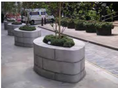
FIGURE 6. HVM PLANTERS SPACED 1200MM APART, WITH MORE THAN 1000MM HEIGHT
