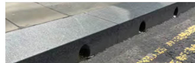
South St David Street – a wide whin kerbstone was specified with apertures to provide a combined kerb and drainage unit.
