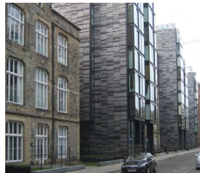
Aluminium: Simpson Loan - Multi-toned anodised aluminium cladding provides a striking and positive contrast to the historic buildings making the distinction between new and old very clear.
