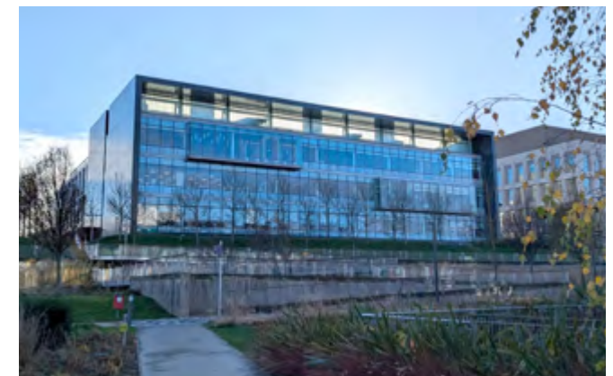
Adaptable laboratory building: Bioquarter - This building was designed to allow different types and sizes of laboratory space and all their associated services to be fitted out and changed over time.
