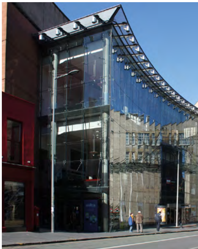
Frameless glazing: Festival Theatre, Nicolson Street - The refined detailing of the frameless glazing helps create a striking modern addition to the street.
