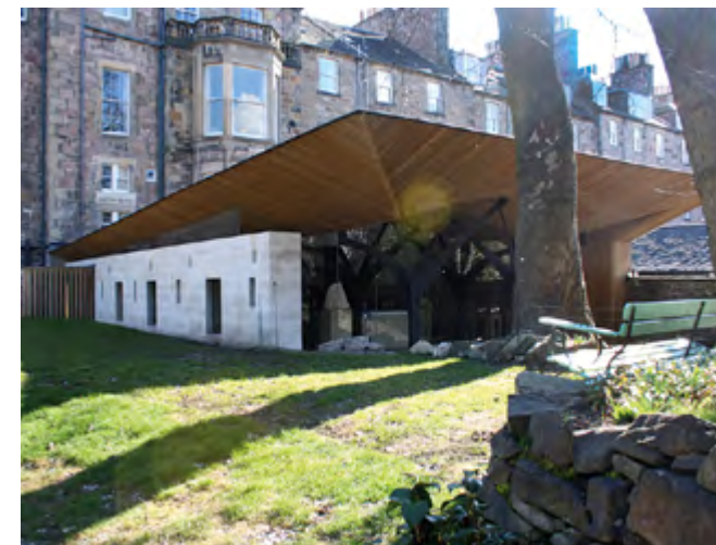
Frameless glazing: Chapel of Saint Albert the Great, George Square Lane - Glazing is used to create the effect of a floating roof on this distinctive Catholic Church.
