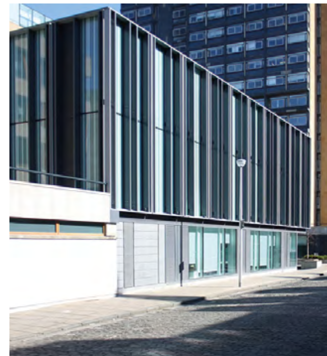
Curtain Walling: Buccleuch Place - The potential offered by glazing systems with variations in the window widths, patterning of the glass and mullion depths is fully taken advantage of here.
