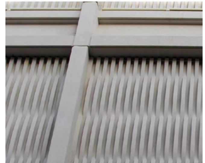
Textures created with concrete - Concrete panels with a textured surface treatment are used on this recent building on Princes Street.
