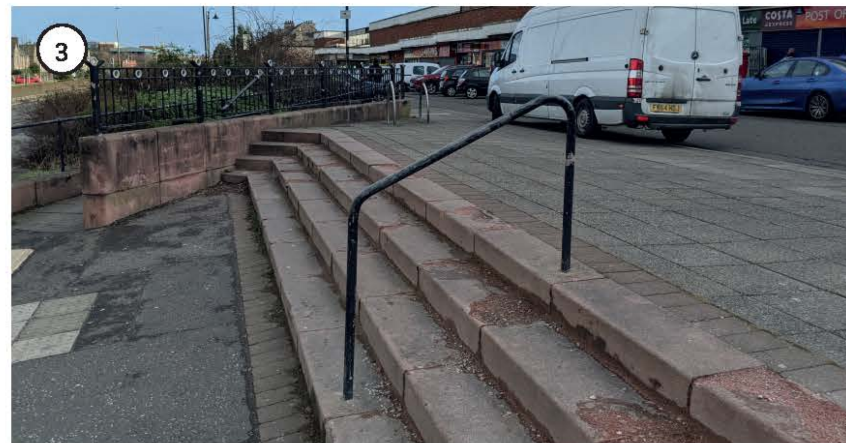
Wide concrete steps in poor repair with only 1 handrail and no tactile paving in place
