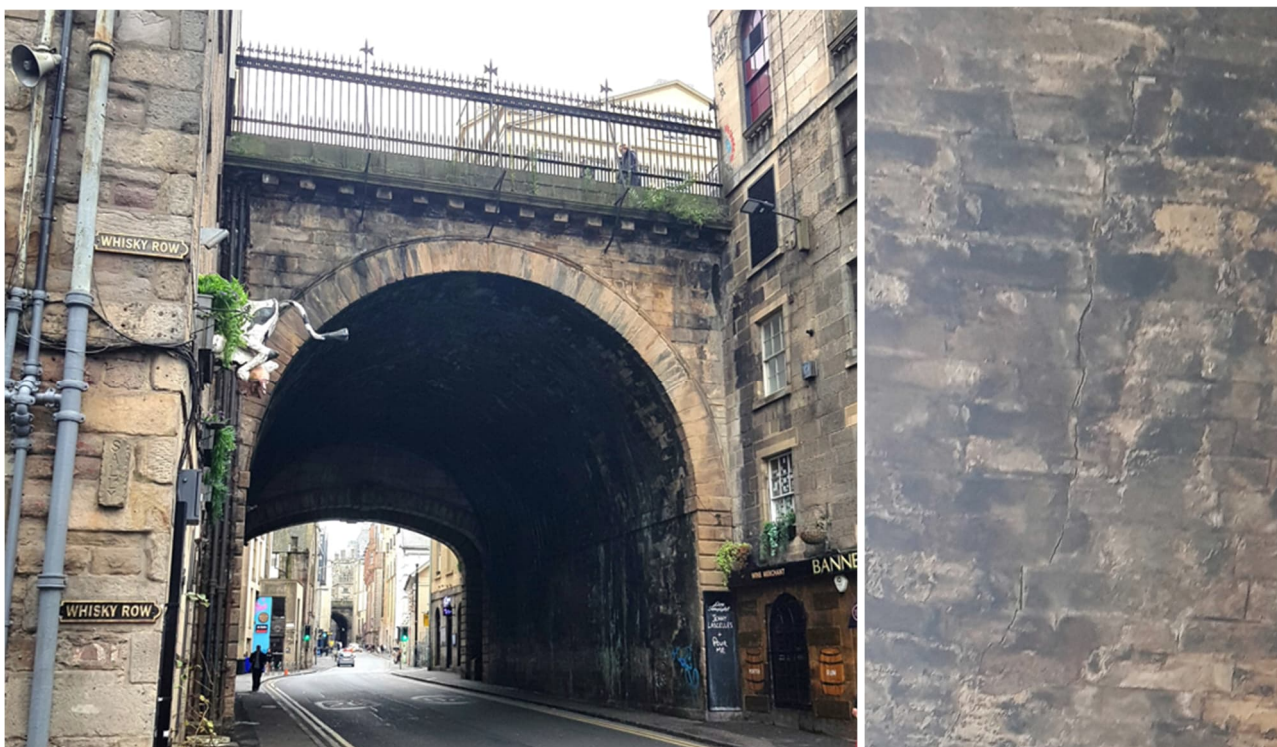
Figure 4.5: Eastern Elevation of the Cowgate Arch (LHS), Longitudinal Arch Crack (RHS)
