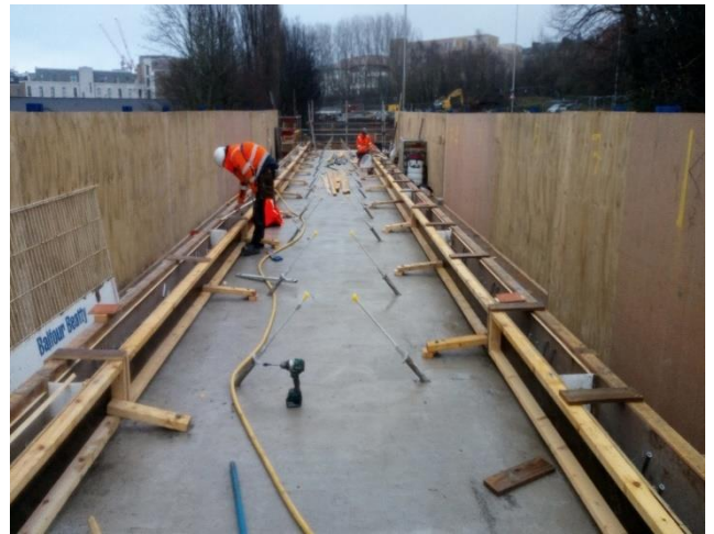
Deck and support structure going in
