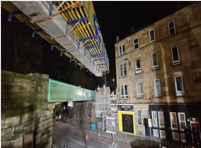
Installation of bridge beam over Dalry Road
