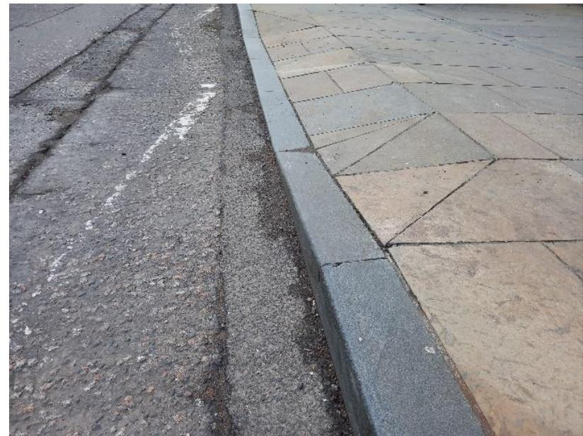
*Photos showing a footway where the full pavement slopes down to meet the carriageway (top photo) and where a steep slope at the carriageway edge has been used to deliver a flatter pavement (bottom photo)*
