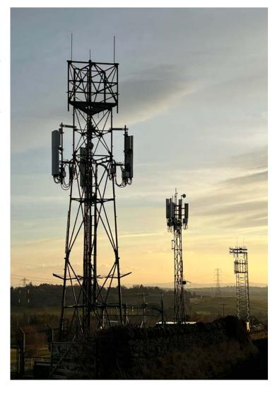
The specific technical infrastructure required for 5G means that sharing is not always possible. While some existing 3G/4G services are provided by existing towers or behind church louvres, the size and weight of 5G infrastructure means that it can often be impractical or impossible to accommodate such infrastructure alongside existing antennas needed for 3G/4G. Therefore, it is often more practicable to install 5G equipment at new sites.
