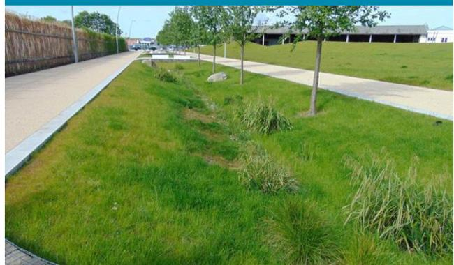
Figure 12. Dry Swale, Dalmarnock Strain Station | SNH
