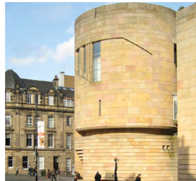
Sculptural and contextual stone cladding - At the Museum of Scotland rigorous and sculptural use of sandstone cladding provides the building with a striking contemporary aesthetic that responds positively to the surrounding historic context. Care needs to be taken with any proposal like this, that the detailing mitigates adverse weathering and staining.
