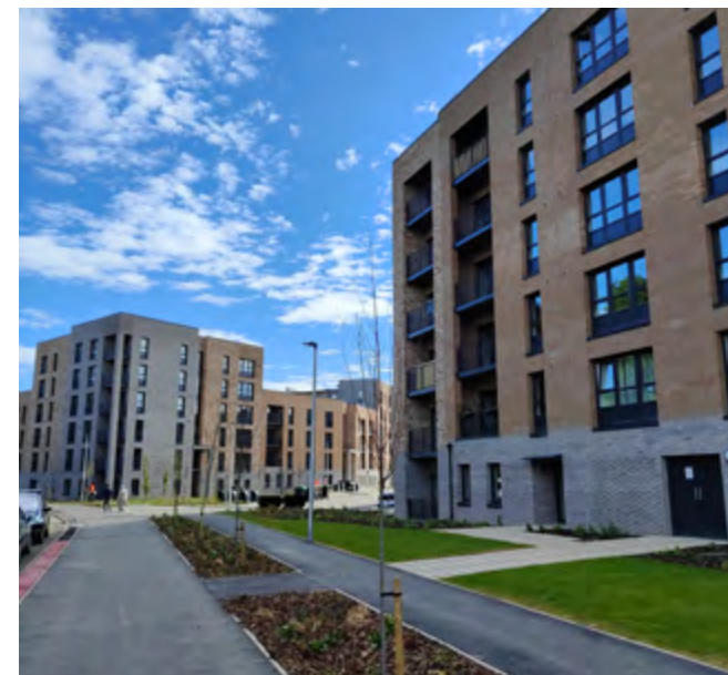
Western Villages, Granton - The new homes at Granton have been constructed using a timber closed panel wall system. These are manufactured offsite, increasing efficiency and reducing waste and transport emissions. The system follows a ‘fabric-first approach’ which improves the thermal performance and reduces the operational emissions of the building.
