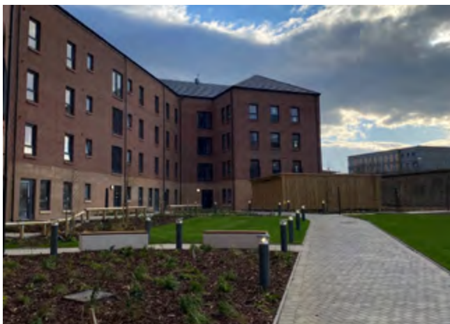
Minimising operational energy emissions - Granton Station View. The development consists of 75 homes for social and mid-market rent. Also on the site are four commercial spaces, communal bike storage and a private courtyard. The project utilised off-site manufacturing to construct a low energy consuming development. This included enhanced building fabric performance, enhanced window specification using triple glazing, a communal energy centre featuring air source and water to water heat pumps, photovoltaic panels and EV charging. The projected operational energy for space heating is an average 19.39 kWh/m 2 /year for the flats.
