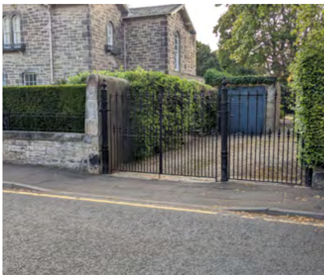
Vehicle crossovers on footways - This vehicle crossover on Greenhill Gardens maintains a level footway suitable for wheeling. Vehicle crossovers (e.g. to access driveways) that slope too steeply can make journeys with a wheelchair or buggy difficult.
