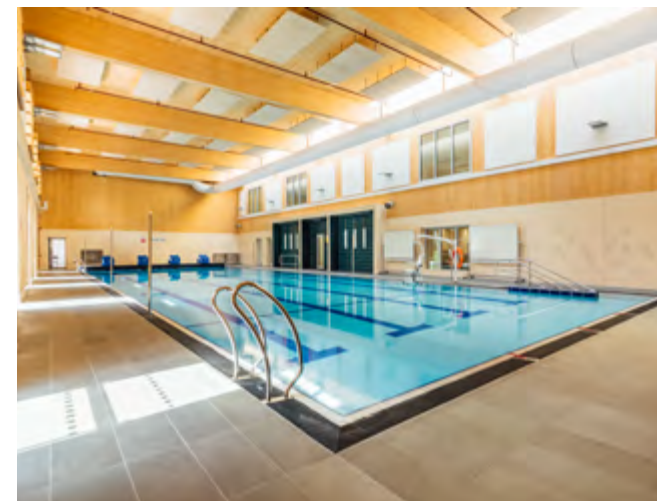
Currie Community High School - One of the first Passivhaus secondary schools in Scotland. The school includes the UK’s first Passivhaus school swimming pool, which was built using a cross-laminated timber and glulam structure.
