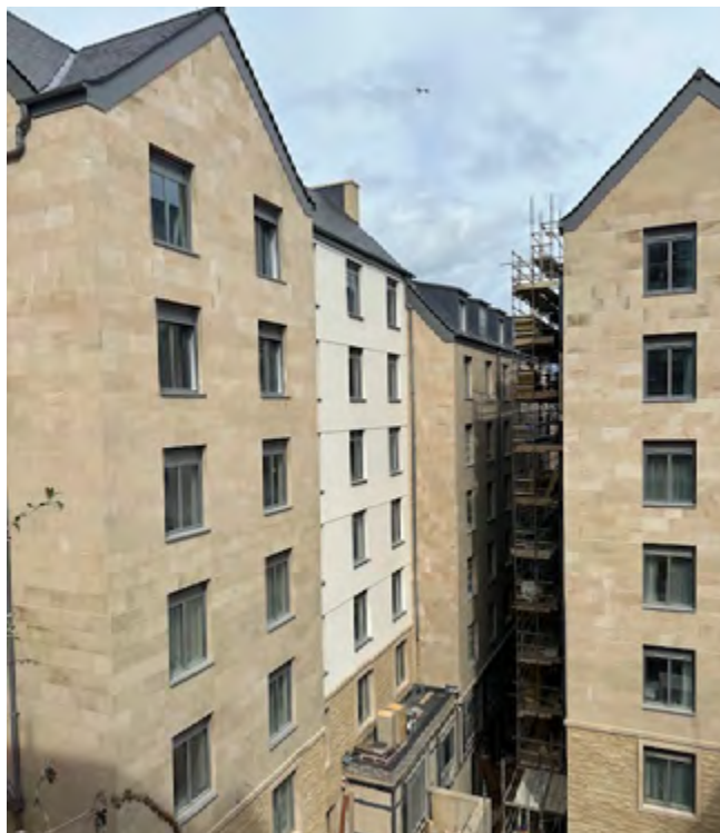
Jury’s Inn, Jeffrey Street - The extension to this hotel uses natural sandstone, a material with high longevity, low maintenance and good potential for future re-use and recycling.
