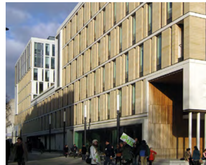
Informatics Forum: Charles Street - Sandstone is built into vertically proportioned panels which are used to order the design of the elevations.
