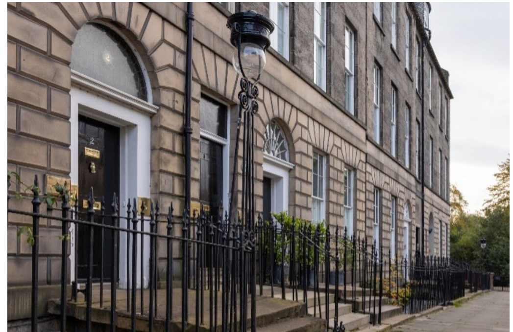
Doorways and fanlights in the New Town Conservation Area.
