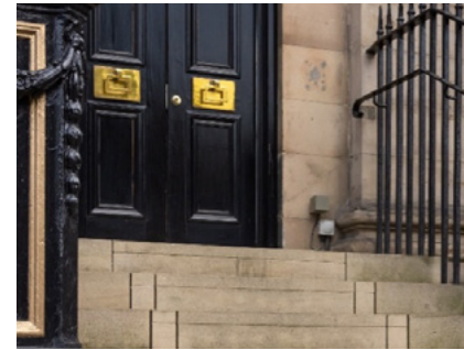
Hidden platform lift at Gleneagles Townhouse Hotel, Category A listed, LB29707, 13/04/1965.
