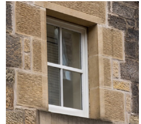
Matching stonework around new window.
