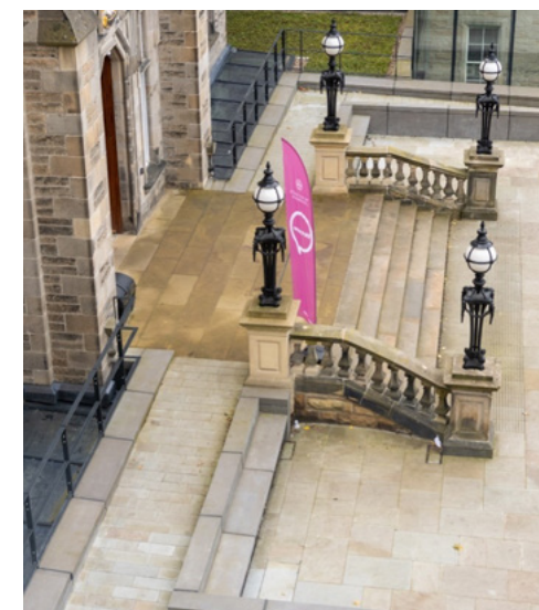
Ramp at Edinburgh Futures Institute. Original stone staircase moved forward to accommodate ramp. Category A listed, LB30306, 31/05/1994.
