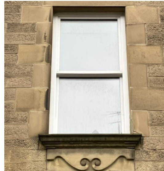
uPVC window closely copying the appearance of a timber sash and case window.
