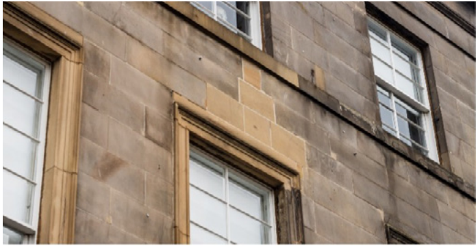
Indent stone repair and matching window details.
