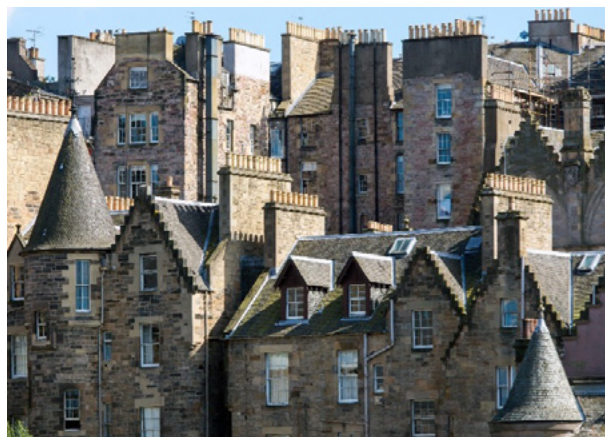
Roofscapes and chimneys from the Old Town Conservation Area.
