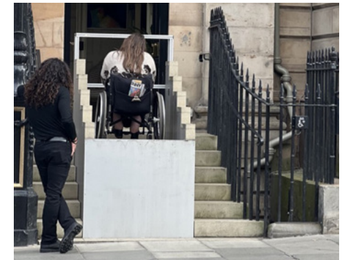
Hidden platform lift in use. Stairs fold back to form the platform and the lift provides level access for the user.
