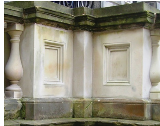
Example of stone repair matching details.
