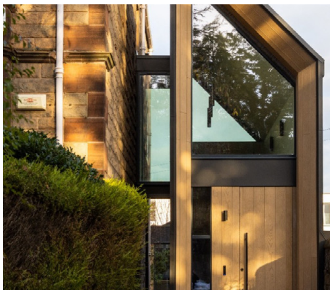
Modern extension designed with a link bridge to an existing opening for minimum fabric removal.
