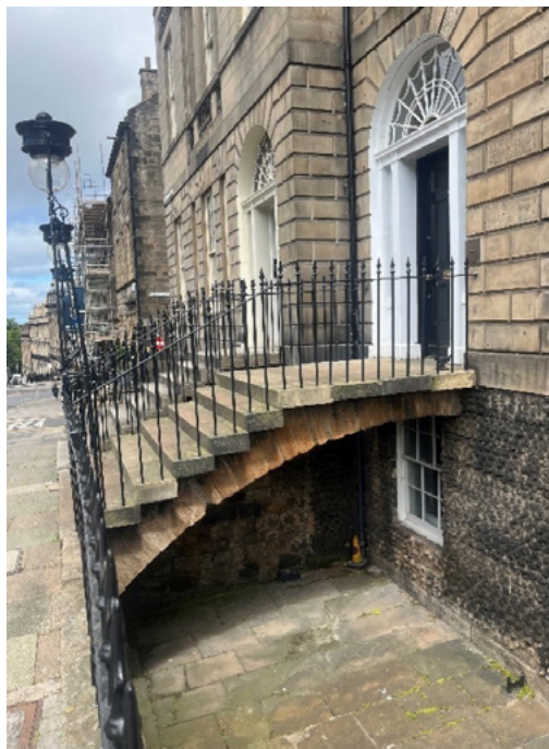
Basement with original stone slabs, and unfilled below platt
