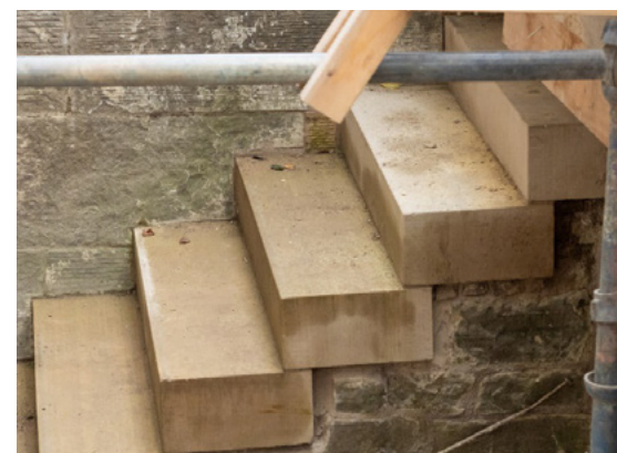
Repair being made to basement stairs.
