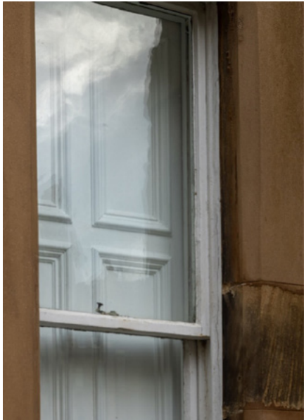
Example of timber window shutters seen from the outside.
