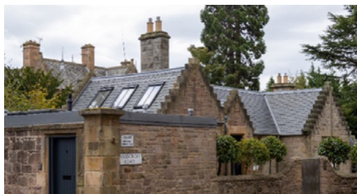
Conversion of a gate house building.
