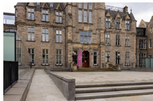
Ramp at Edinburgh Futures Institute. Original stone staircase moved forward to accommodate ramp. Category A listed, LB30306, 31/05/1994.
