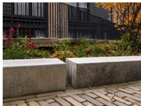
Public realm seating with channel to allow drainage into adjacent rain garden.
