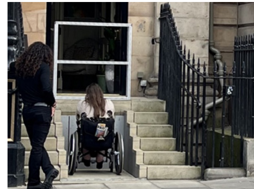
Hidden platform lift in use. Stairs fold back to form the platform and the lift provides level access for the user.
