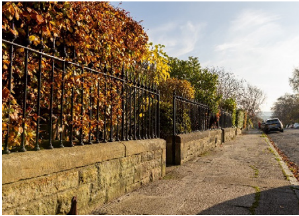
Traditional low boundary wall with railings.
