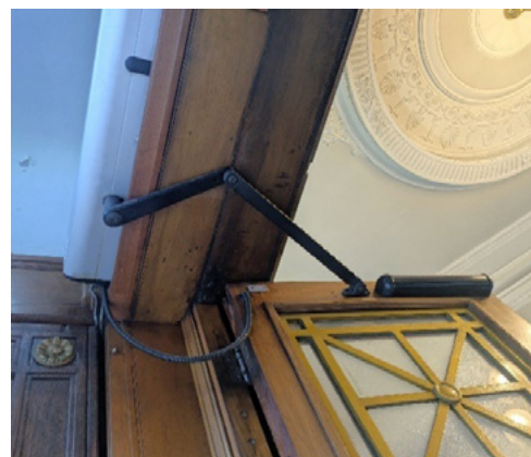
Door opening mechanism.
