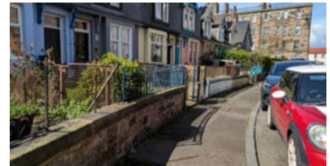
Characteristic stone walls and railings
