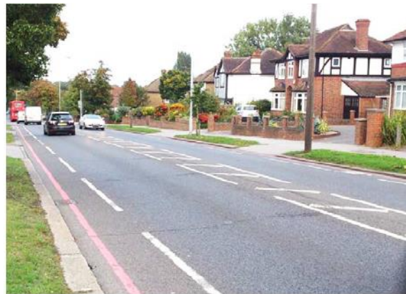
Centreline removal & Cycle lane widening Before & After TfL, 2014, Centreline Removal Trial.
