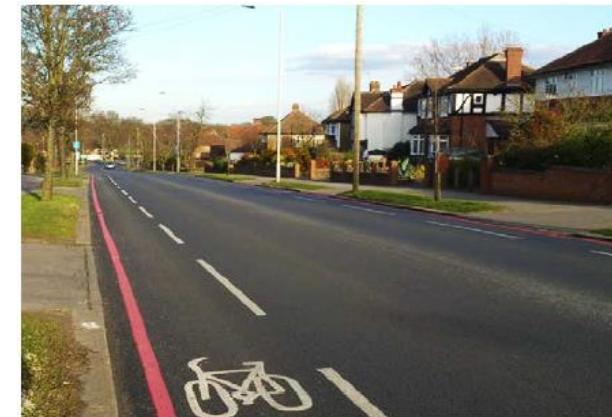
Centreline removal & Cycle lane widening Before & After TfL, 2014, Centreline Removal Trial.
