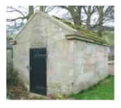
Swanston Road Water House: Single storey, single-bay rectangular, stone-built water house with stone flagged roof, category B listed, dated 1761. The water house is built around a water gauge which was used to supply water to the city from Swanston. The gauge was used for measuring and regulating the flow of water from Hare Burn and the water was conveyed in wooden pipes and linked to the supply at Comiston.
