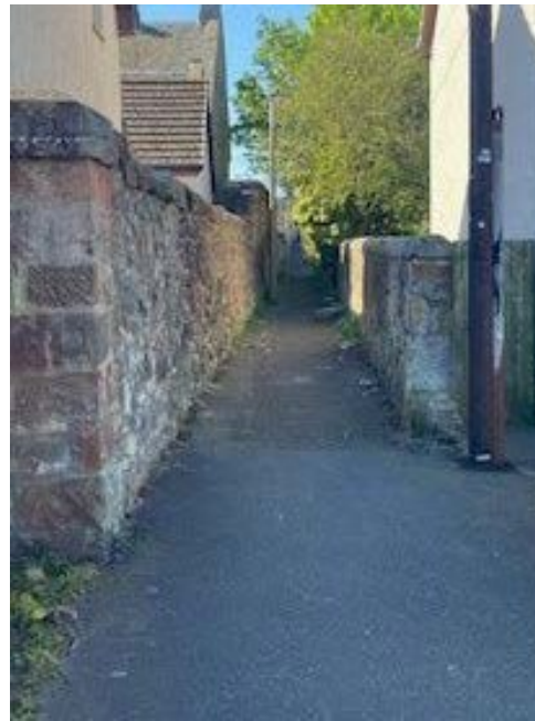
The Vennel from Hawthorn Place
