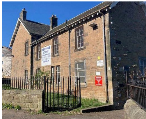
Former convalescence home Newtoft Street
