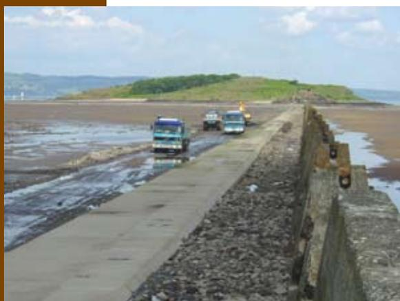
There is also a row of concrete stanchions, which were erected as part of the Firth of Forth defences during World War II and were originally linked by concrete shuttering, the remains of which can be seen strewn around their bases.
