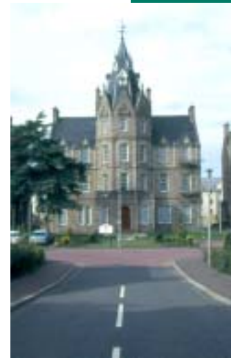
original baronial style building
