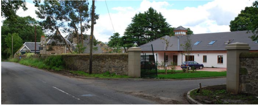
Caern House with Steading buildings beyond
