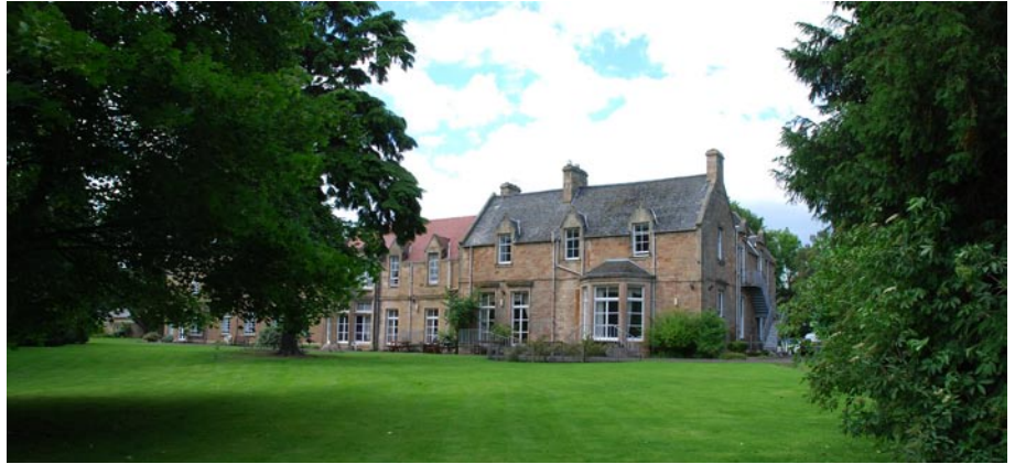
Kirklands House south front
