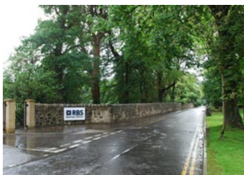
West gate and boundary wall
