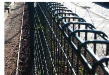
On low metal mesh fences (this example 1.5m), the top should be rolled for safety. Black powder coated mesh good for townscape setting.
