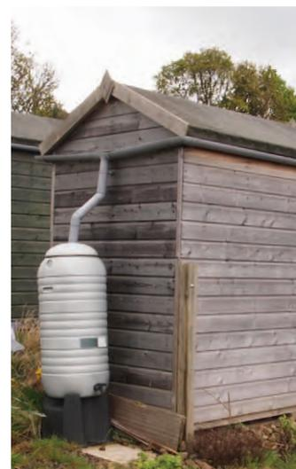
This proprietary water butt system connects to the gutters. Works on double pitch roofs, 200L butt shown. Bridgend Farm, Edinburgh
