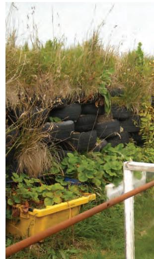
A perimeter windbreak at an allotment site on Shetland: recycled tyres backfilled with soil. These can be planted to create a green wall
