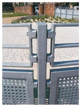
The perforated panels were selected to allow some airflow through the screen and to reduce the turbulence that would be created by solid elements. Galvanised steel panels were used as a durable, costeffective solution.
