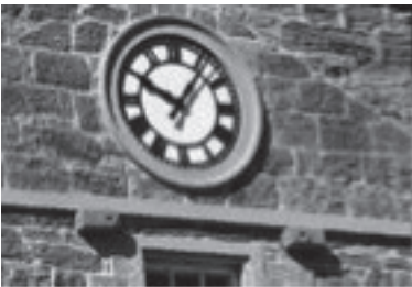
Figure 6 - Swift boxes installed on Culzean Castle, A Listed Building, Ayrshire
