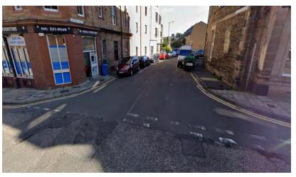
Photo of the junction after the width has been reduced and tactiles and dropped kerbs have been installed
