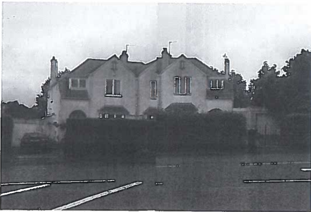
Photos 08 and 09 – 5 & 7 Corbiehill Road (both with single storey, flat roof garage)
