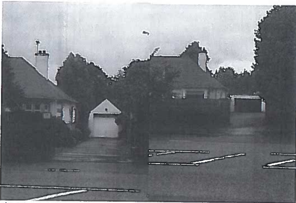
Photos 03 & 04 – 68 (single storey, pitched roof garage) & 64 Hillhouse Road (single storey, flat roof garage)
